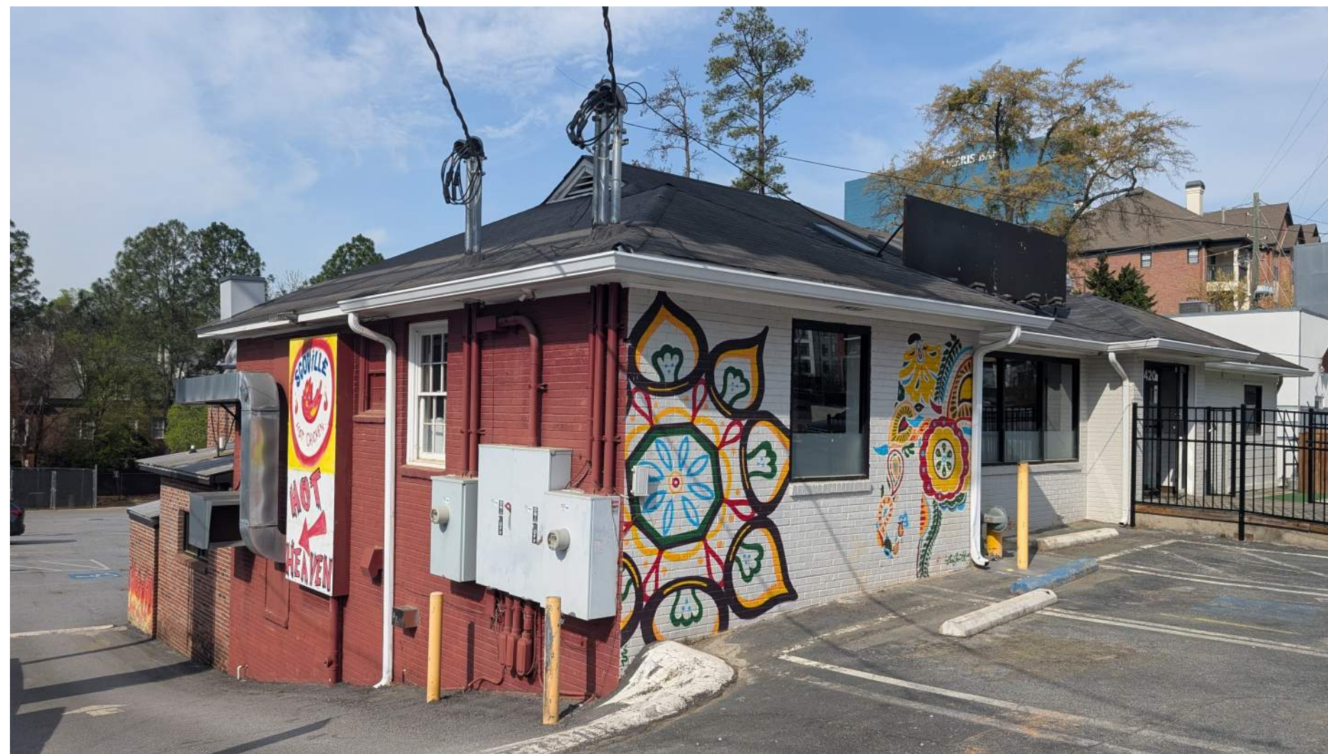
6 EXIST. PHOTO - NORTH EAST CORNER AD4.01 N.T.S.
