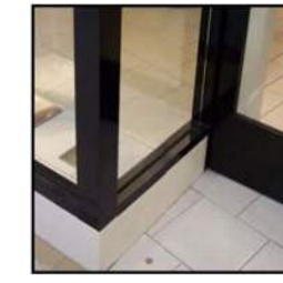
ALUMINUM STOREFRONT SYSTEM FINISH: ANODIZED BLACK
