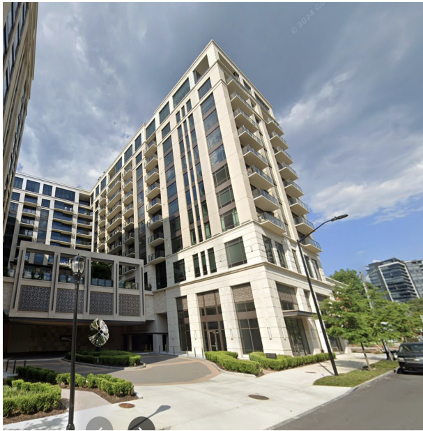
EXISTING WEST FACADE
