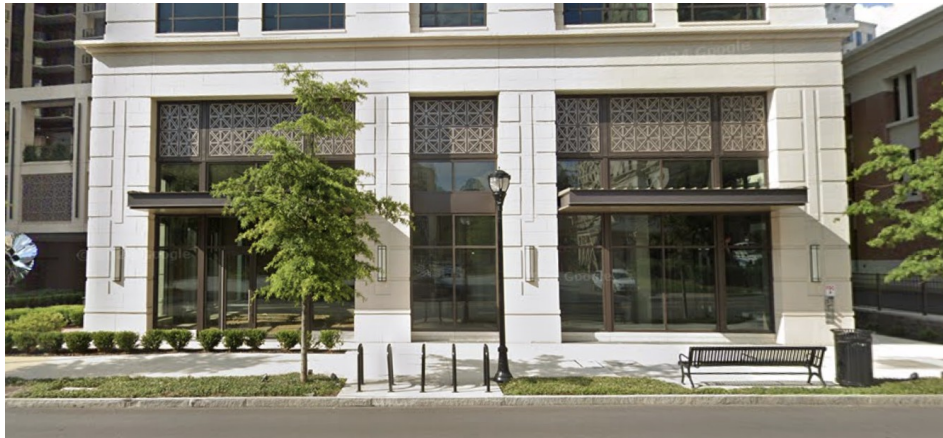
EXISTING SOUTH FACADE West Paces Ferry Frontage
