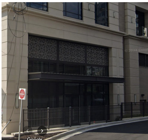
EXISTING EAST FACADE
