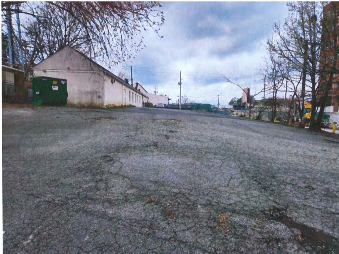
2. Rear and North Side of Existing Building
