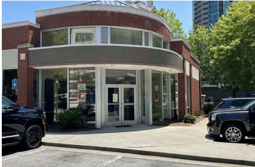
Existing Main Entry Close-Up
