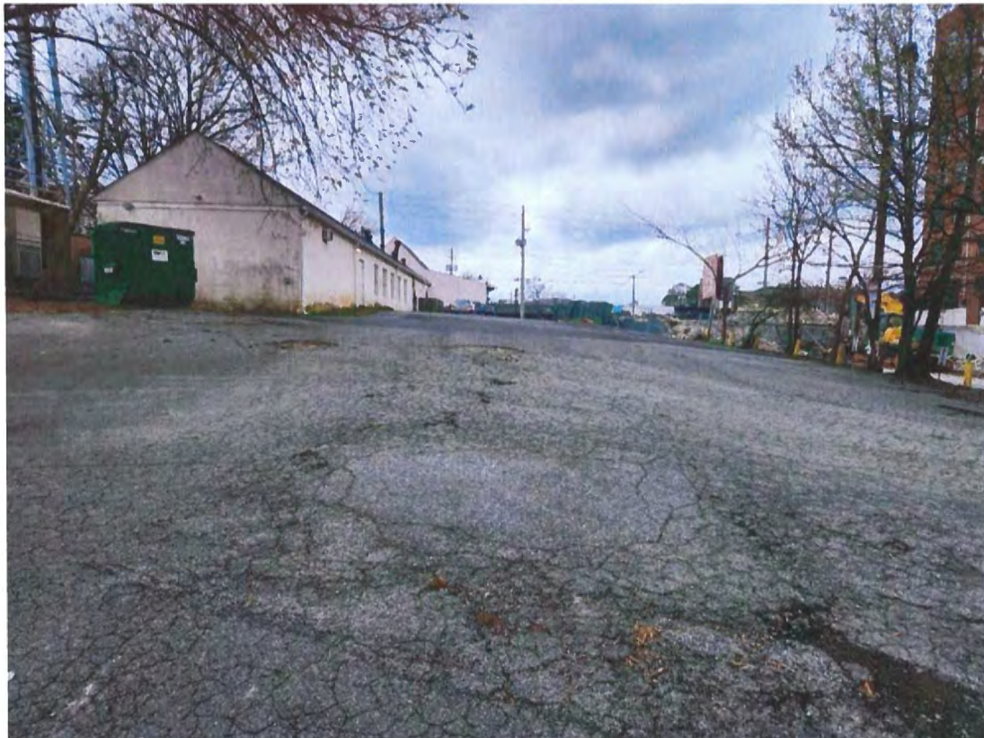
2. Rear and North Side of Existing Building
