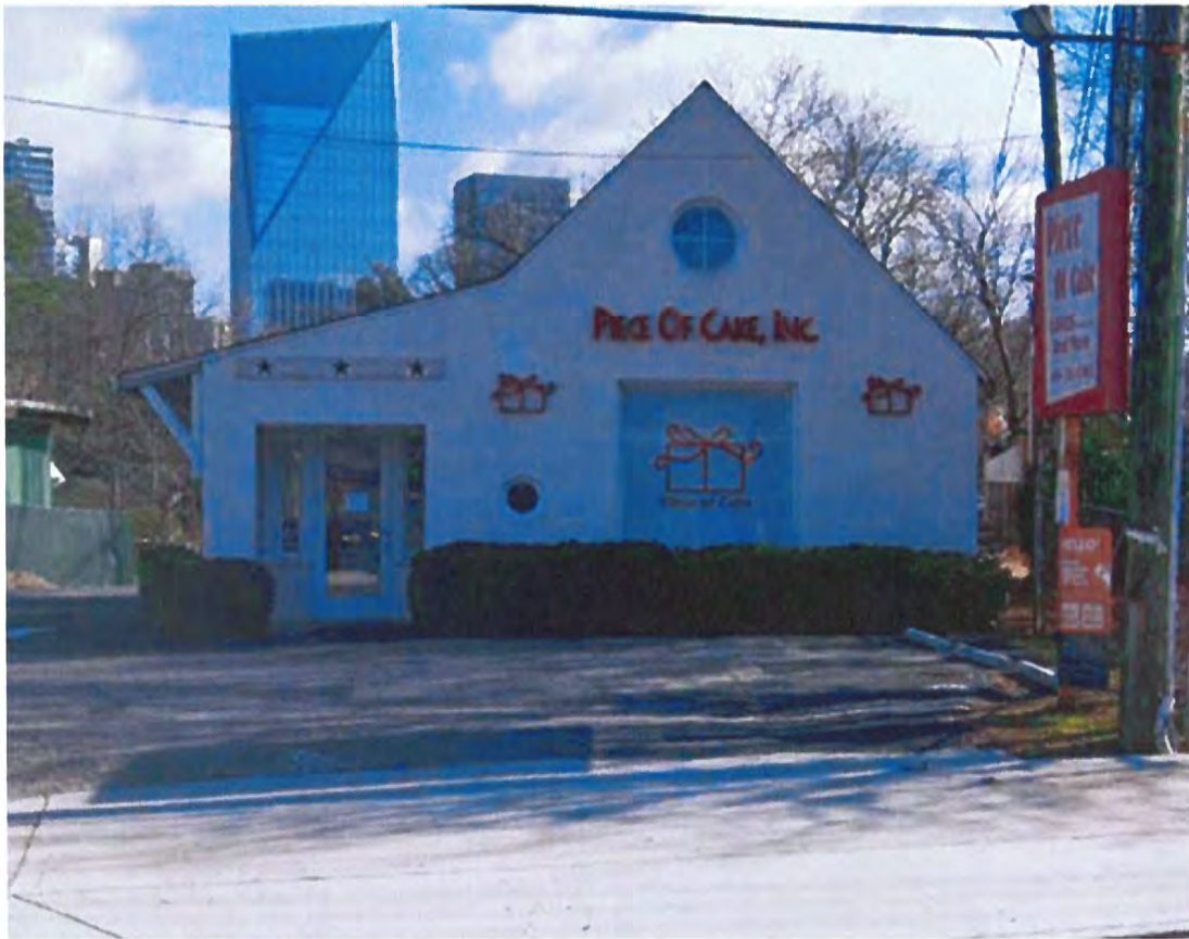
1. Front of Existing Building
