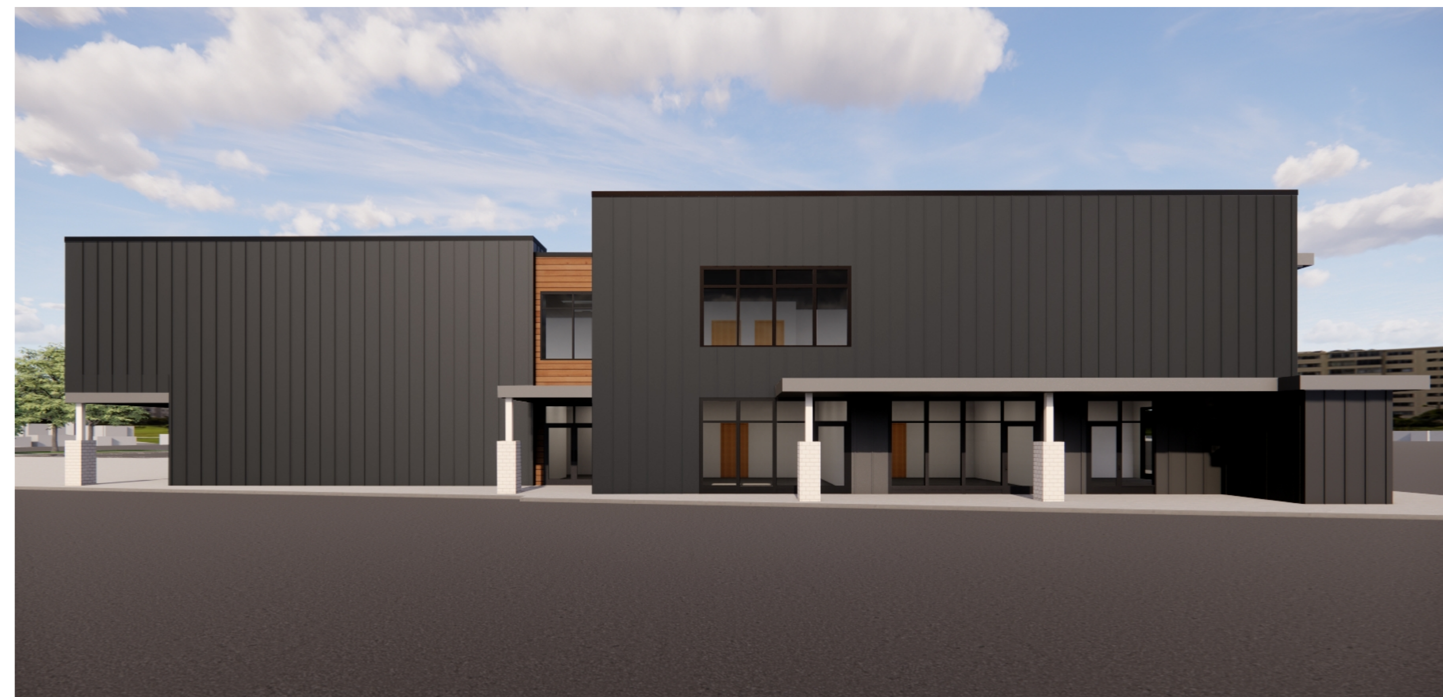
SIDE (VIEW TOP OF SITE)
