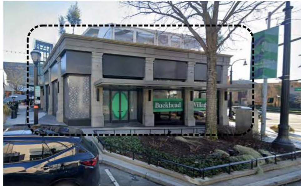
EXISTING - BUCKHEAD AVENUE
