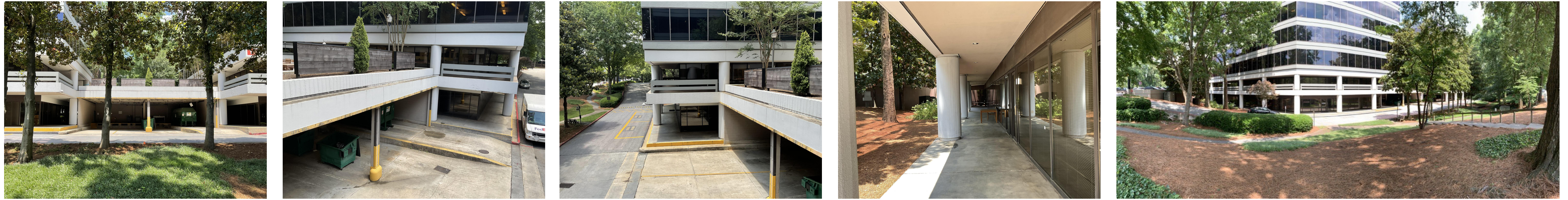
EXISTING CONDITIONS PHOTOS
