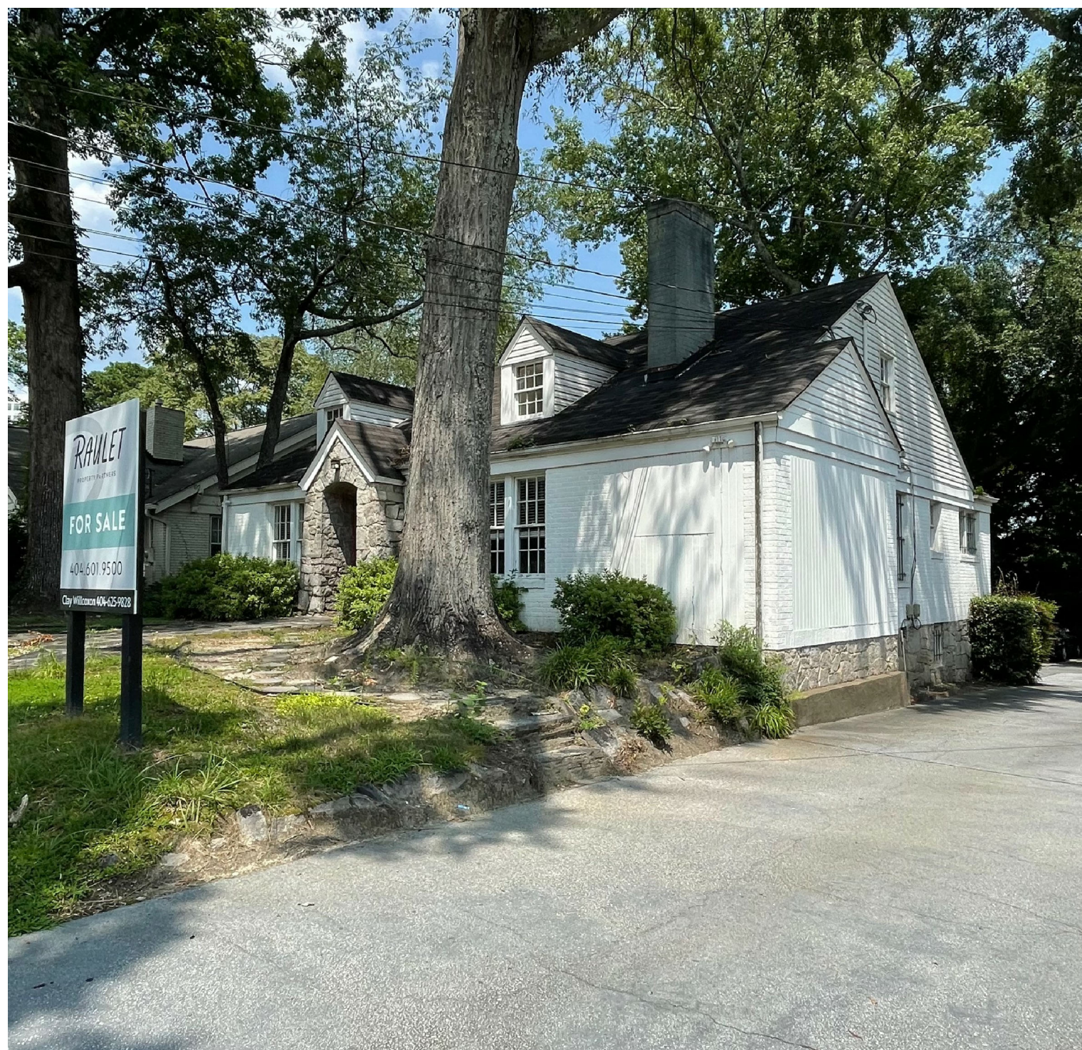
2 EXISTING STREET FRONT PHOTO A-1 NOT TO SCALE
