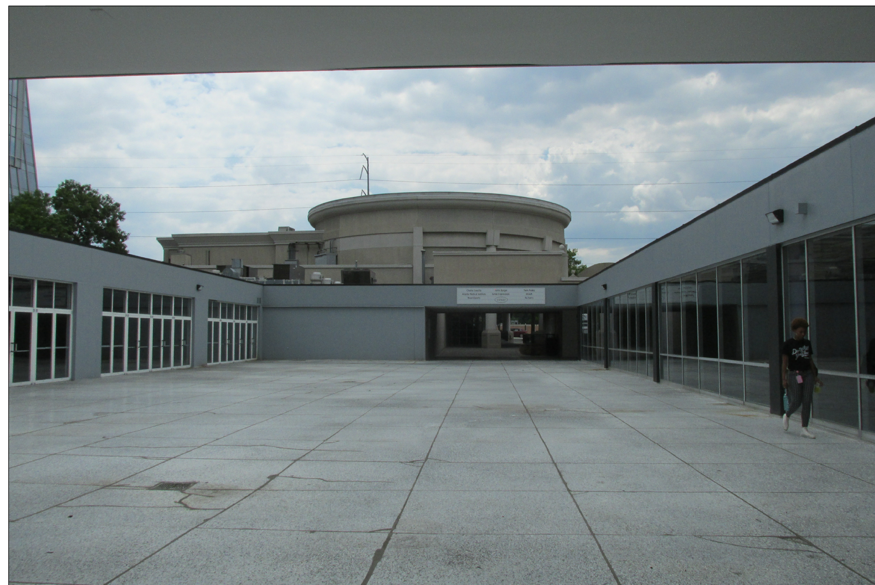
2 VIEW LOOKING WEST - PIEDMONT ROAD IS ON THE OTHER SIDE OF THE ROUND SHAPED ELEMENT
