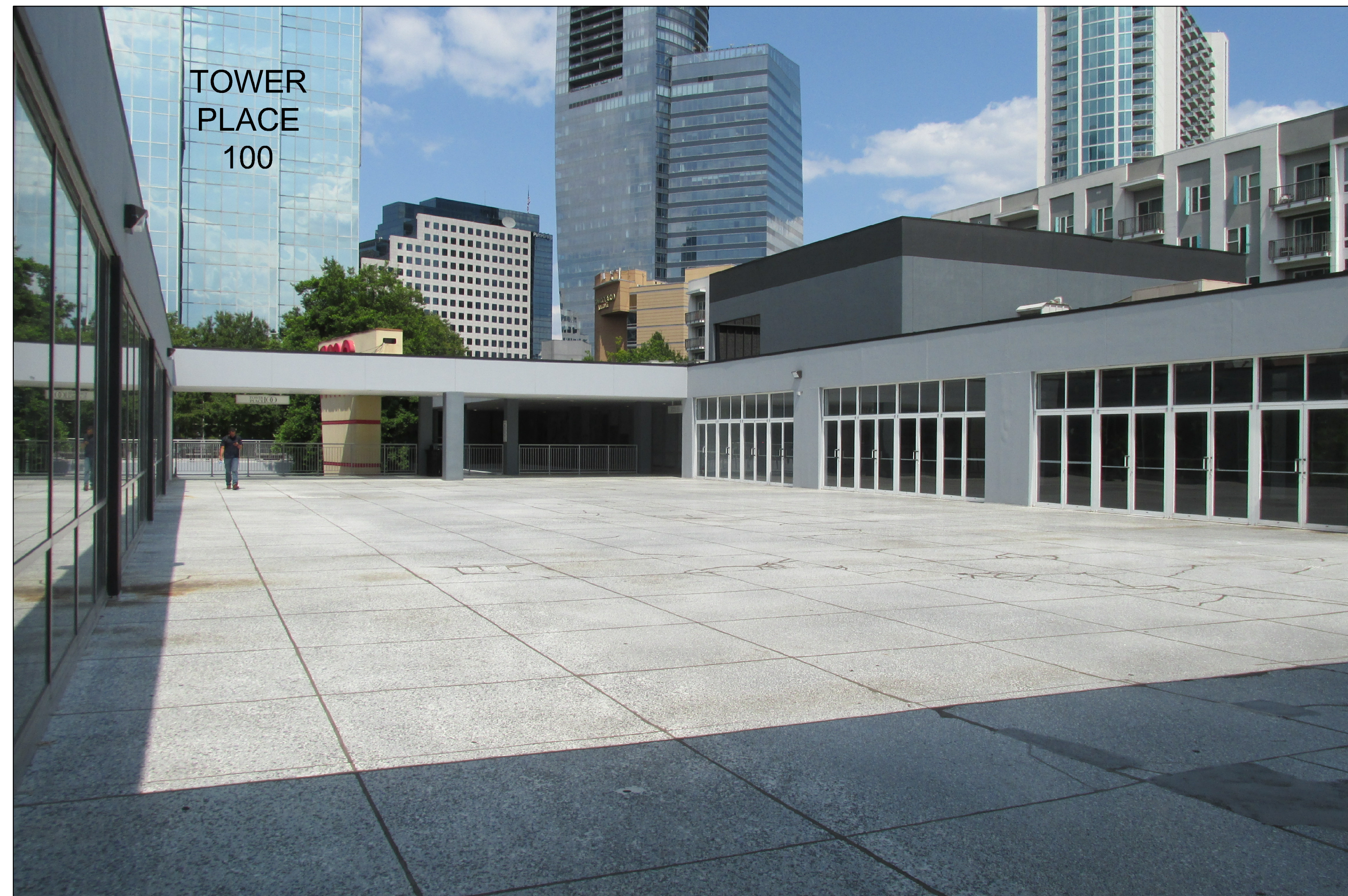
1 VIEW LOOKING EAST AT THE EXISTING COURTYARD (APPROXIMATELY 60'-0" WIDE X 120'-0" LONG)
