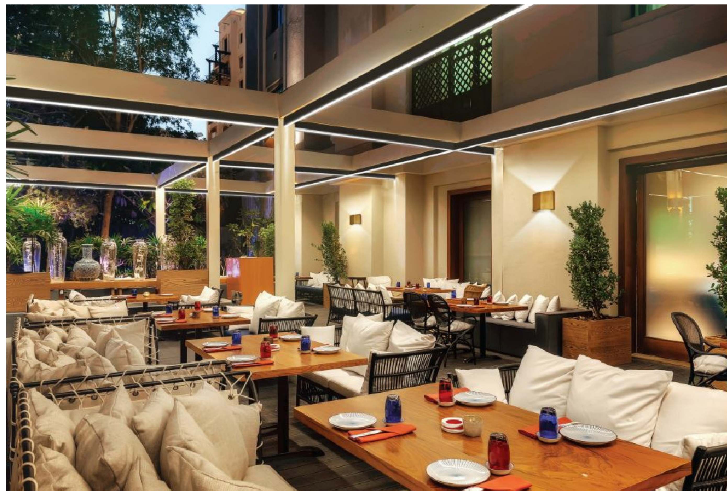
A EXAMPLE OF SURFACE MOUNTED LIGHTING AT UNDERSIDE OF TRELLIS FRAMING MEMBERS
