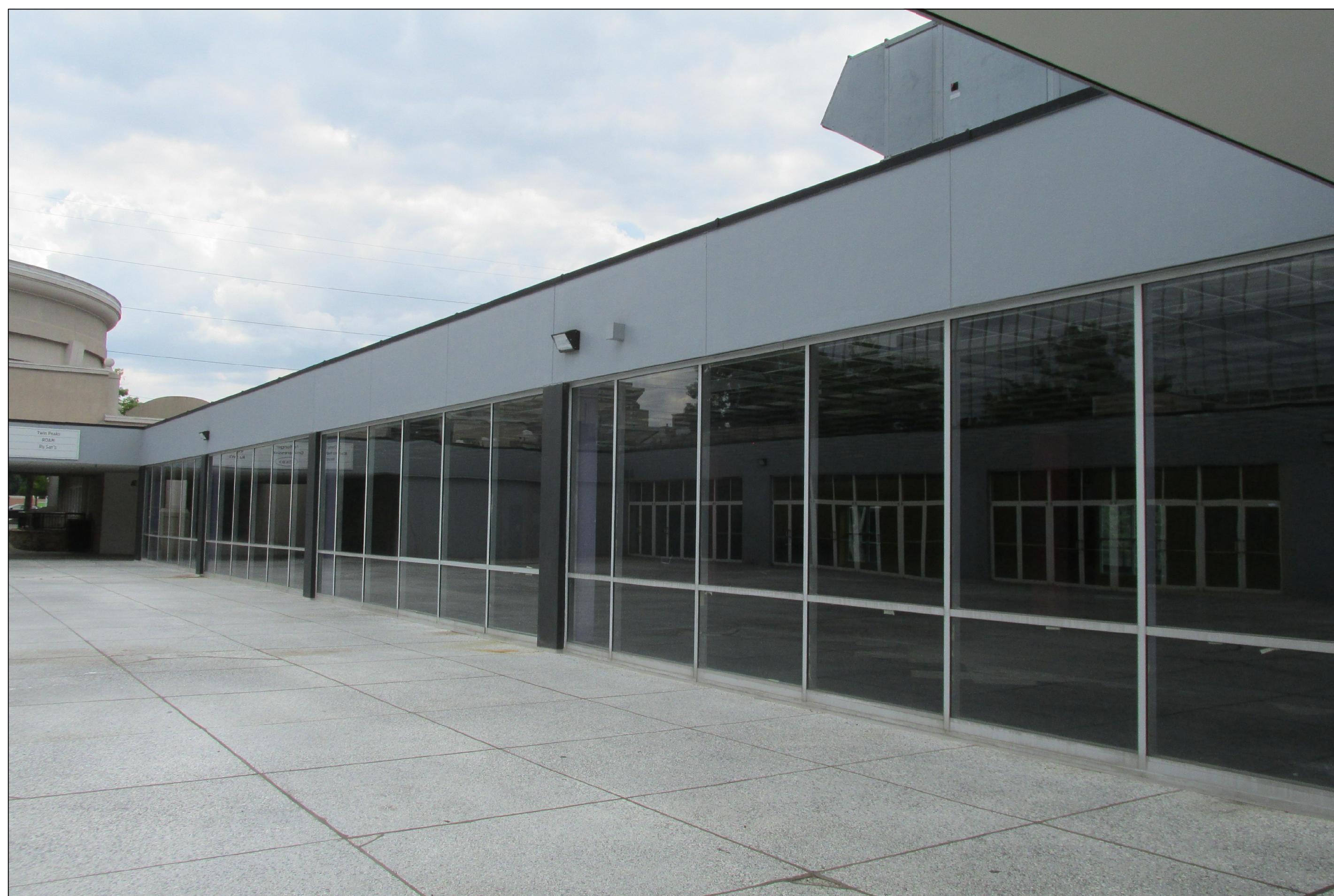
4 VIEW LOOKING EAST AT EXISTING STOREFRONT ON SOUTH SIDE OF COURTYARD
