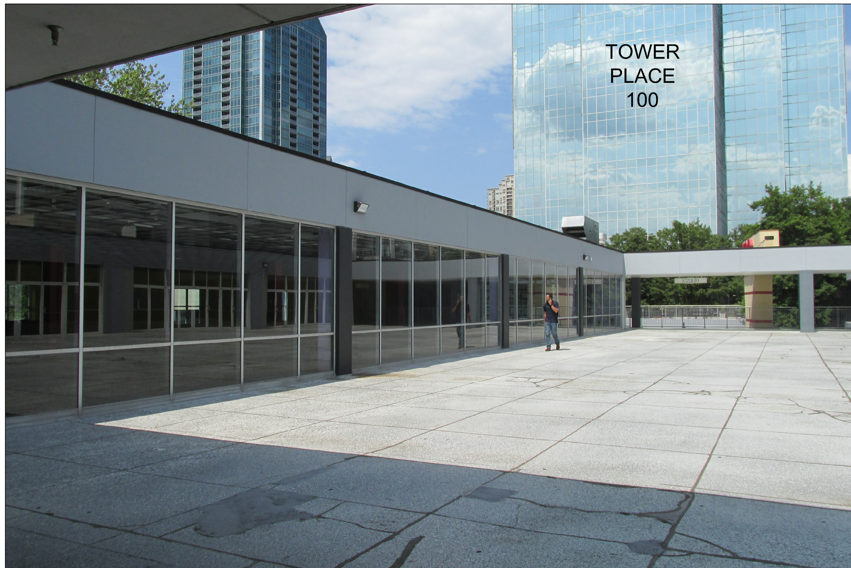
3 VIEW LOOKING EAST AT EXISTING STOREFRONT ON NORTH SIDE OF COURTYARD
