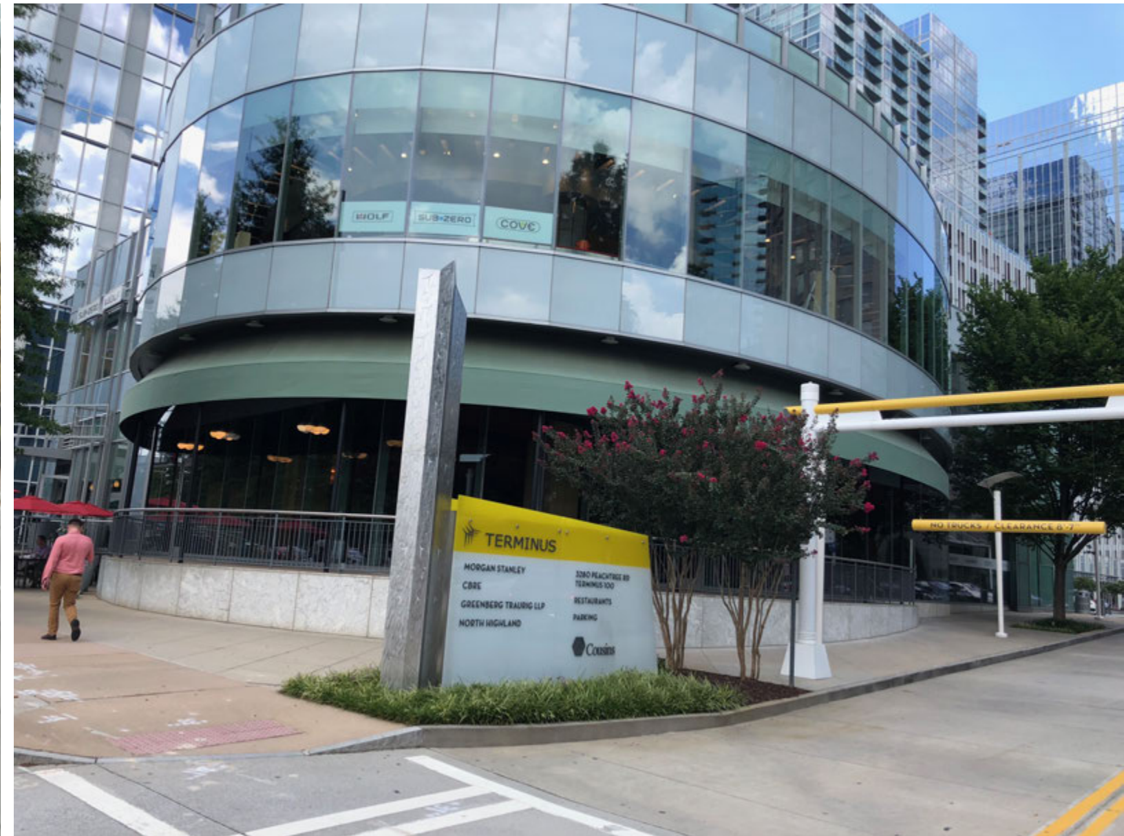
2 EXISTING SITE REFERENCE IMAGE
