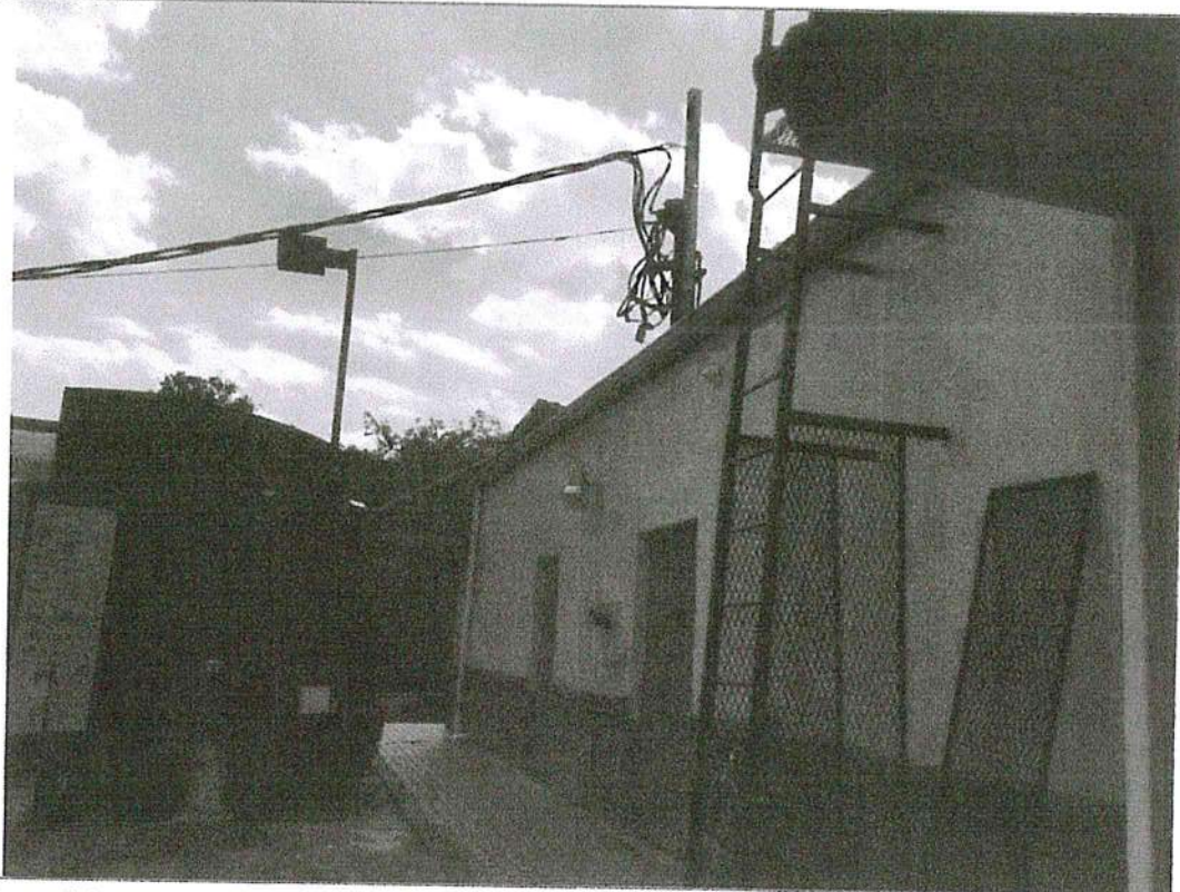
Rear of the Building
