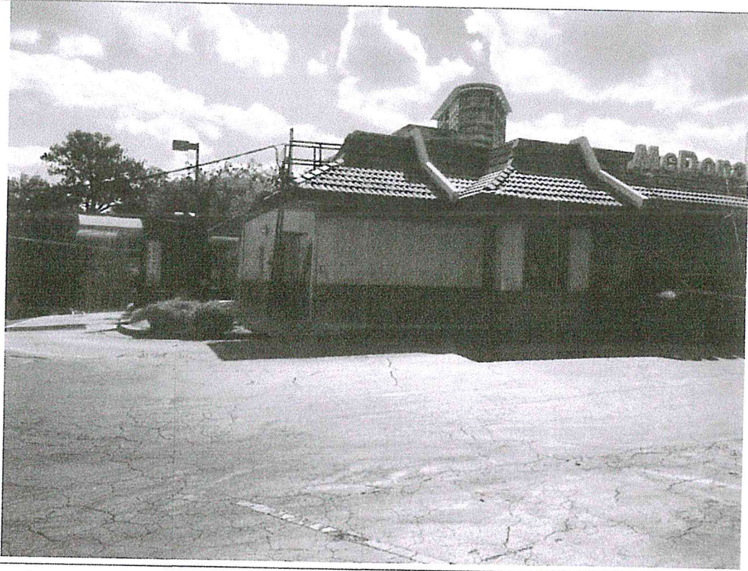
DT and rear of the building
