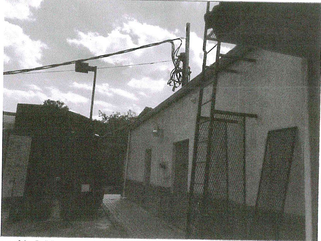
Rear of the Building
