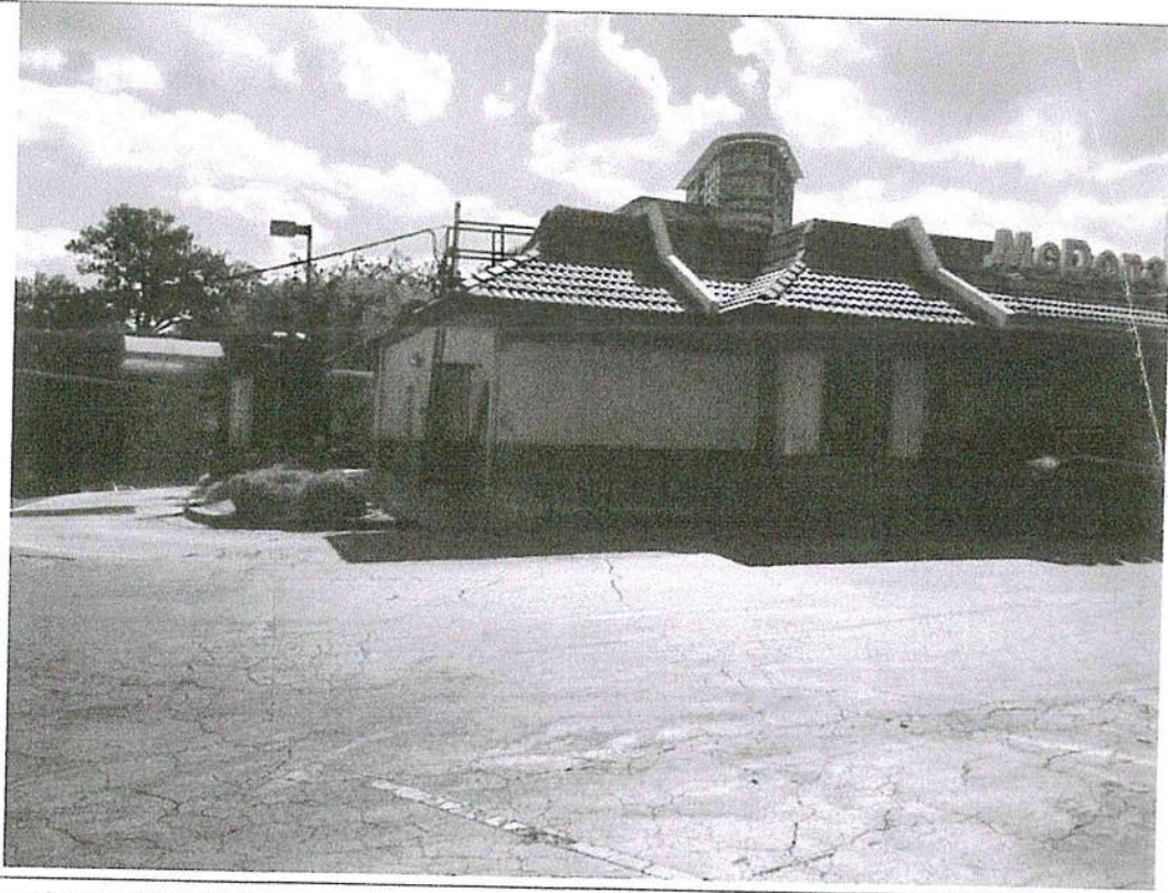
DT and rear of the building
