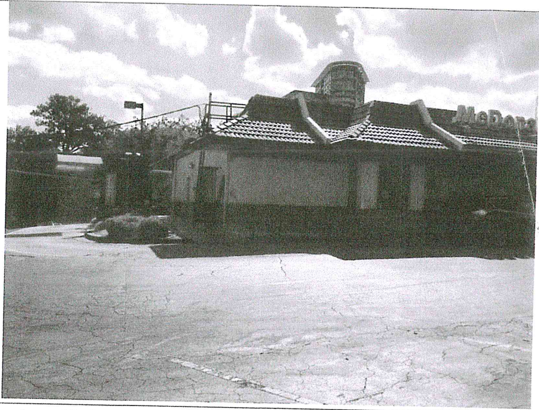
DT and rear of the building
