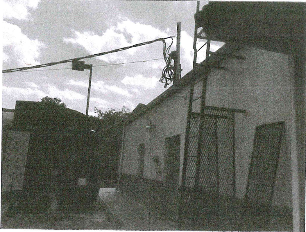
Rear of the Building
