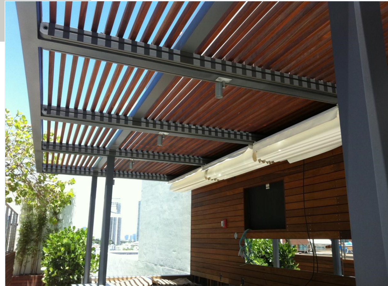
PRECEDENT PHOTO OF ALUMINUM CANOPY WITH SAPELE WOOD FIXED LOUVERS AND RETRACTABLE CANVAS AWNING
