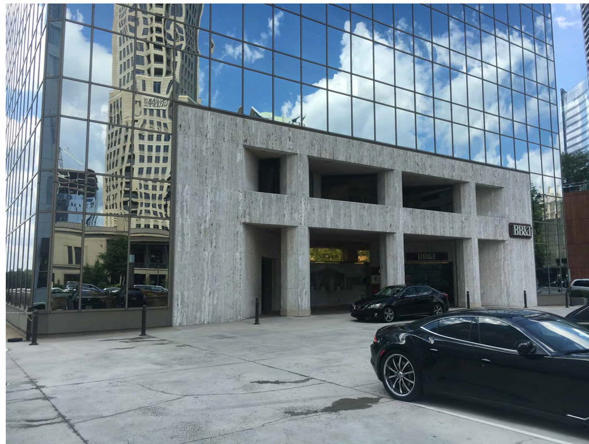
EXISTING FACADE PHOTO
