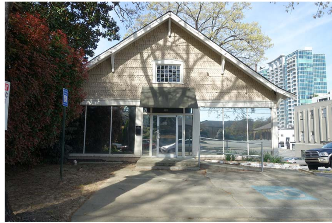
1 FRONT OF EXISTING BUILDING G0.4
