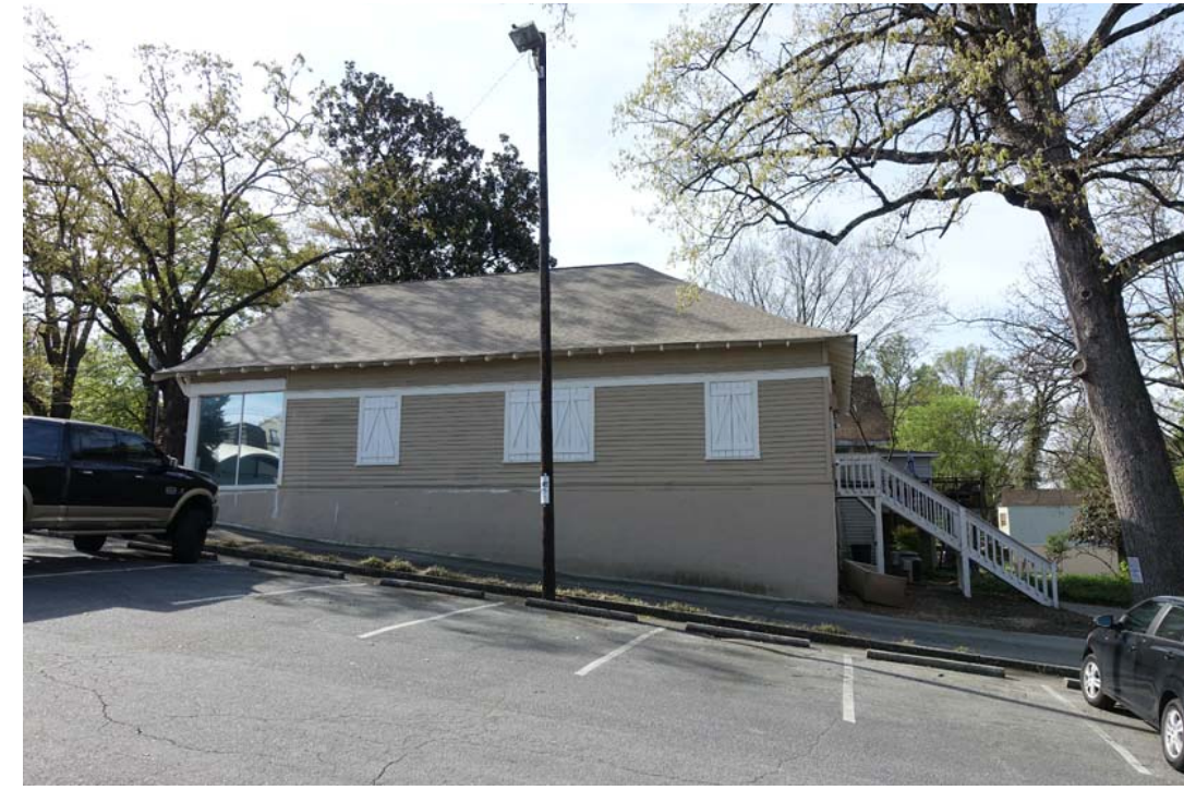
2 SIDE OF EXISTING BUILDING G0.4
