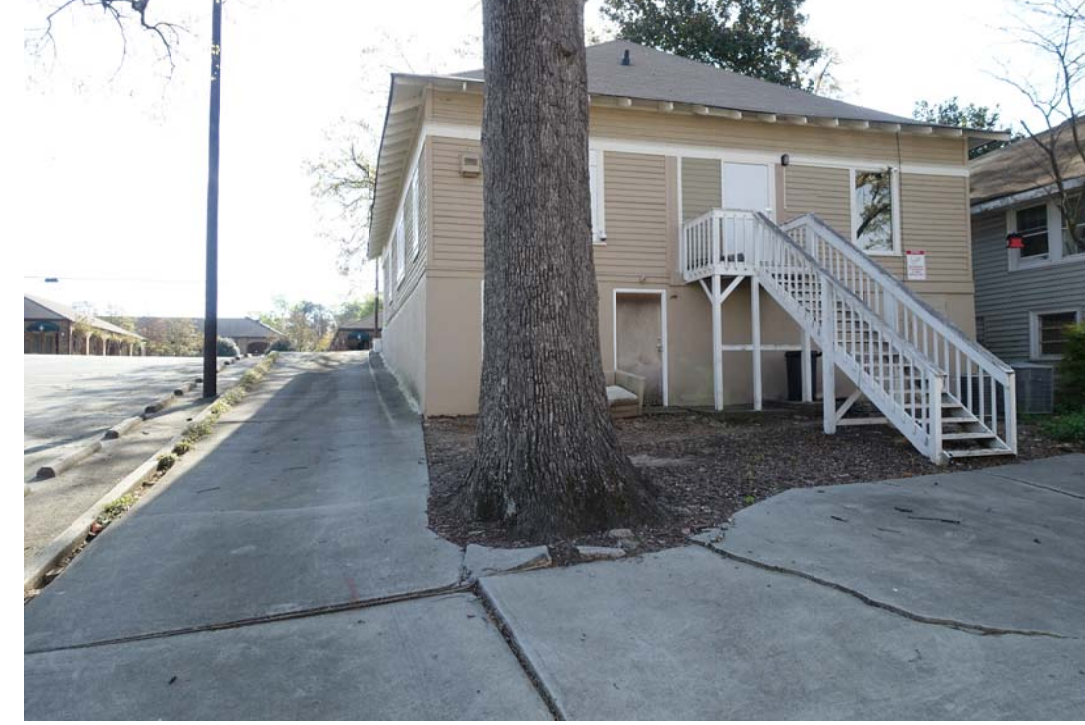
3 BACK OF EXISTING BUILDING G0.4
