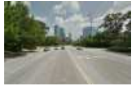
01/06 PIEDMONT STREET- SOUTH APPROACH
