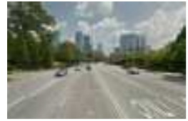
02/06 PIEDMONT STREET- SOUTH APPROACH
