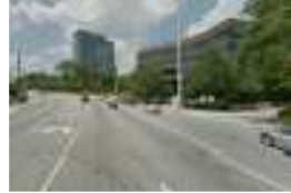
04/06 PIEDMONT STREET- NORTH APPROACH
