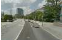
02/06 PIEDMONT STREET- NORTH APPROACH
