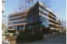
05/06 PIEDMONT STREET- NORTH APPROACH
