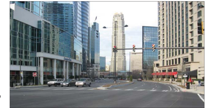
Completed Phase I Peachtree Road Complete Streets project
